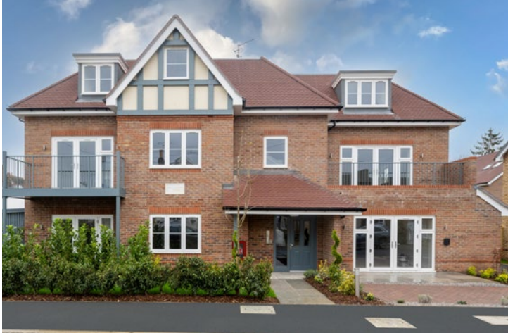
Ashcroft Place, Staines-upon-Thames
